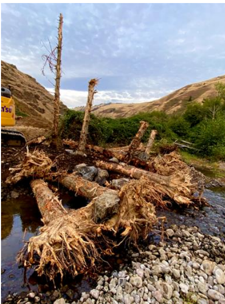
Figure 9. Rectification bank treatment and overhead cover implemented 2024, RM 5.2.
