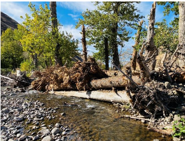
Figure 27. ELJ Bank Structure near RM 4.1 provided quality fish habitat uplift.
