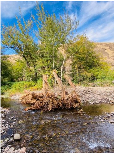
Figure 9. Rectification bank treatment and overhead cover implemented 2024, RM 5.2.
