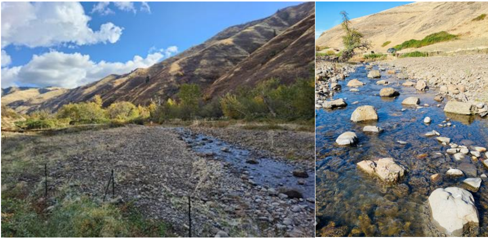
Figure 32. North Fork Walla Walla River RM 4.9 before construction condition.
